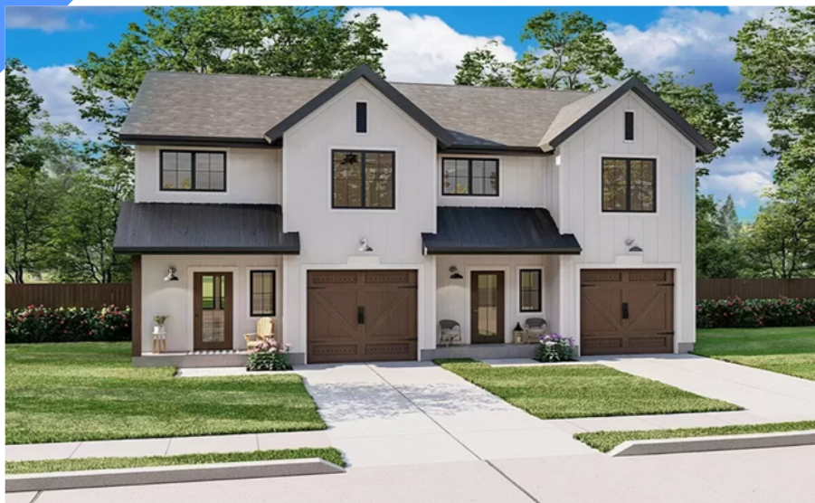
An example of a duplex. Image Credit: Architectural Designs.
